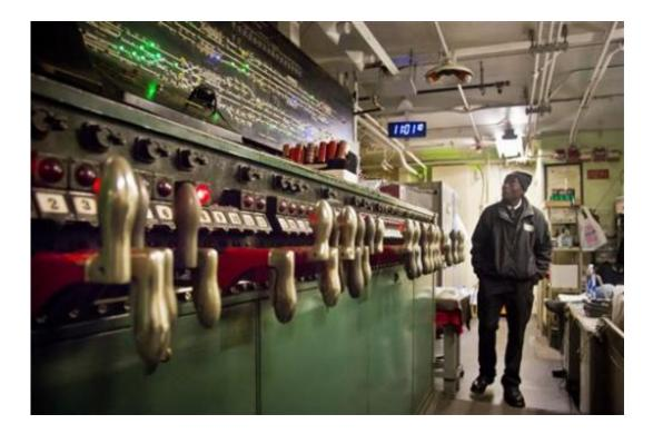
In this Dec. 16, 2014 photo, MTA train service supervisor Tweh Friday monitors a subway interlocking switch and signal control board, at the 4th Street MTA Supervisory Tower in New York. The 1930s technology of switches and relays requires a human operator to use hand levers to manually route trains and keep them separated at safe distances. (AP Photo/Bebeto Matthews)
