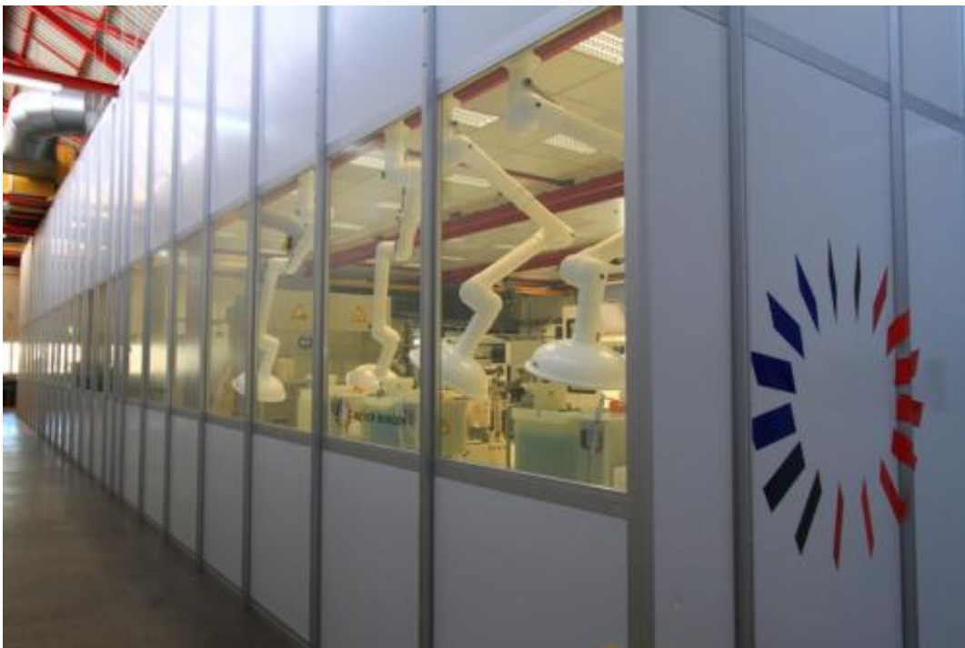
Pilot plant - SwissInno-HJT
