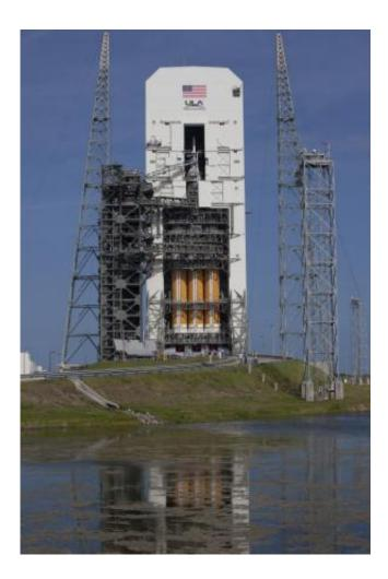
With access doors at Space Launch Complex 37 opened, the Orion and Delta IV Heavy stack is visible in its entirety inside the Mobile Service Tower where the vehicle is undergoing launch preparations. Credit: NASA/Kim Shiflett
