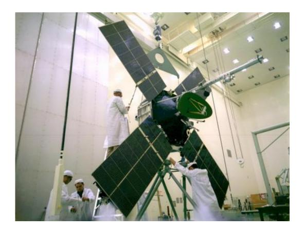
The Mariner 4 spacecraft was assembled by engineers and technicians at the Jet Propulsion Laboratory in Pasadena, California. It is seen here being prepared for a weight test on Nov. 1, 1963. Credit: NASA/Jet Propulsion Laboratory
