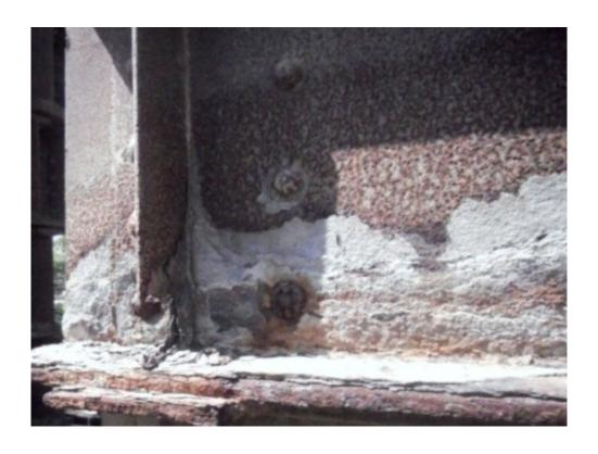
Actual damage on steel structures, alongside output damage modes of steel girder ends from the model developed by Sasaki and his team at Tokyo Tech.
