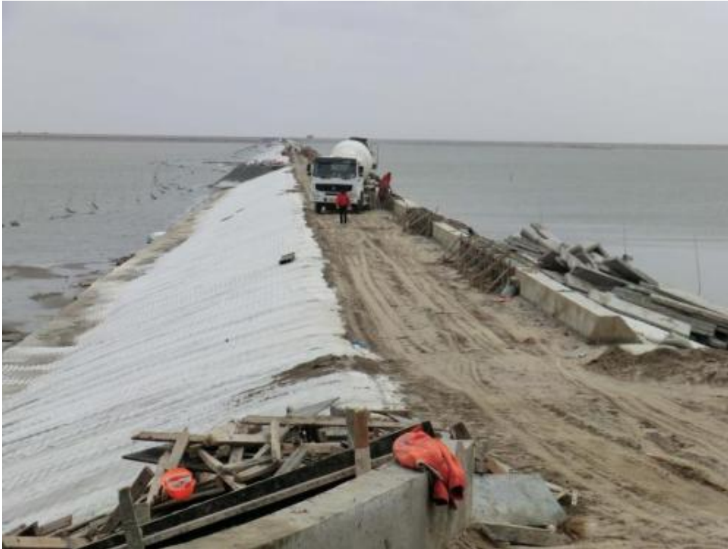
A seawall that is being built in China's coasts. Credit: David Melville and Ying Chen
