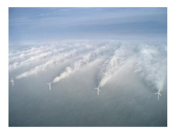
Wind parks produce their own air circulation dynamics. First row turbines get more wind than those in the middle. They also produce vortices that affect the performance of downstream turbines. Learning software can reduce these effects by optimizing rotor speeds and blade angles.
