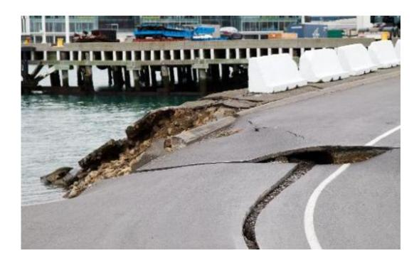
Large cracks caused by an earthquake on July 21, 2013 pictured at the Port Wellington Container terminal
