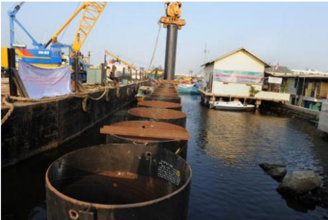
A wall of giant iron reinforcement pipes is installed during the construction of the Jakarta sea wall, October 9, 2014
