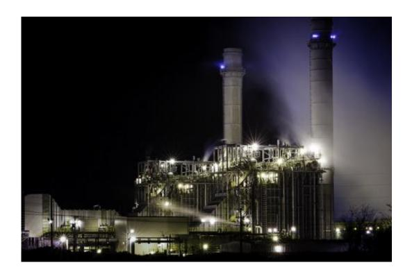
The Hermiston Generating Plant in Umatilla County, Oregon, resides nine miles south of the Columbia River. This 474 MW natural gas power plant generates electricity for consumers, steam for an adjacent potato processing plant, and contributes gray water to farmers. Credit: Scott Butner
