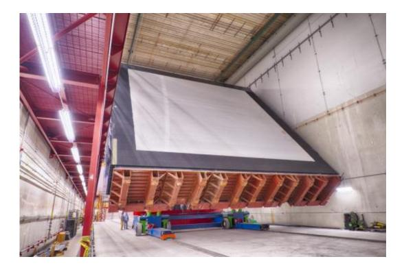
The massive pivoting machine moves one block of the NOvA far detector across the hall in Ash River, Minnesota, to connect it with the rest of the detector. Each block measures 50 feet by 50 feet by 6 feet, and was assembled from PVC modules crafted by University of Minnesota students. Credit: Fermilab.
