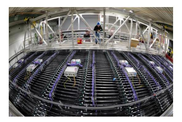
A view across the top of the NOvA far detector in Ash River, Minnesota. Electronics that make up part of the data acquisition system are installed along the top and sides of the detector. The far detector measures roughly 200 feet long, 50 feet high and 50 feet wide, and is made of PVC filled with a scintillating oil. Neutrino interactions inside the detector create light, which travels up fiber optic cables to the banks of computers. Credit: Fermilab.
