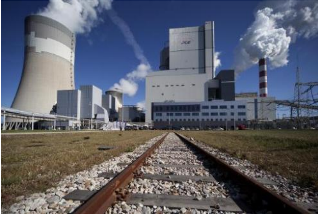
Poland's Belchatow coal-fired power plant on September 28, 2011
