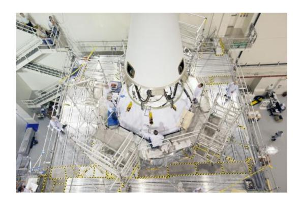
The launch abort system is lowered by crane for installation on the Orion spacecraft for Exploration Flight Test-1 inside the Launch Abort System Facility, or LASF, at NASA's Kennedy Space Center in Florida. Credit: NASA/Cory Huston
