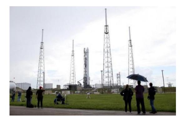
SpaceX Falcon 9 rocket carrying a Dragon supply ship is seen surrounded by lightning protection system towers as it is being prepared for the launch on September 20, 2014, in Cape Canaveral, Florida
