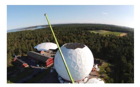
The 20-metre radio telescope at Onsala Space Observatory, is getting a new lease of life thanks to an upgrade of its protective radome.
