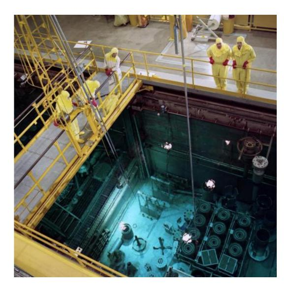
The High Flux Isotope Reactor vessel at Oak Ridge National Laboratory resides in a pool of water illuminated by the blue glow of the Cherenkov radiation effect.
