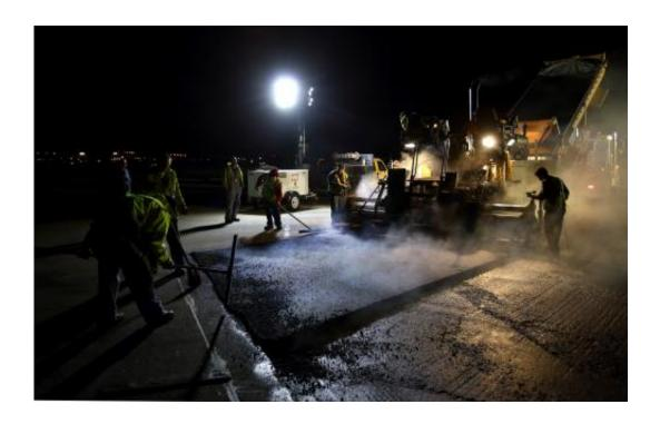
Developed by Sandia National Laboratories and several industry partners, the fuel cell mobile light offers a cleaner, quieter alternative to diesel-powered units. As seen here (top center), the system has been used by airport construction personnel at San Francisco International Airport and in other applications. Credit: Dino Vournas
