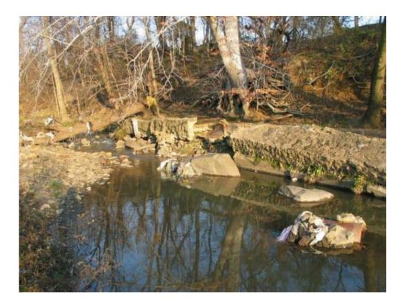
Eroding stream banks and aging sewer lines contribute to evolving water pollution problems in cities. In this photo from Baltimore, Maryland, a sewage pipe that was originally placed in a stream bed developed leaks, and is now surrounded by a concrete casing. Credit: Tamara Newcomer Johnson, University of Maryland
