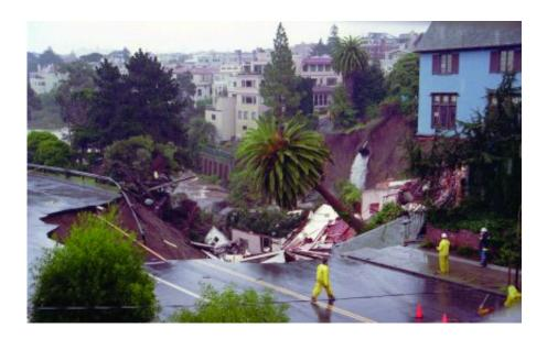
The collapse of corroded concrete sewer pipes can cause major infrastructure damage, such as this sinkhole created in San Francisco. Credit: AP via AAP/George Nikitin
