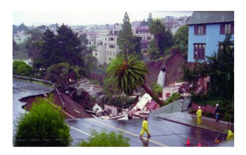
The collapse of corroded concrete sewer pipes can cause major infrastructure damage, such as this sinkhole created in San Francisco. Credit: AP via AAP/George Nikitin
