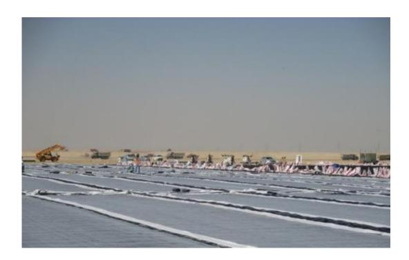
The researchers' material, shown being installed at a site in the Middle East, combines sodium bentonite clay and polymers to create a substance that can withstand industrial waste. Credit: CETCO
