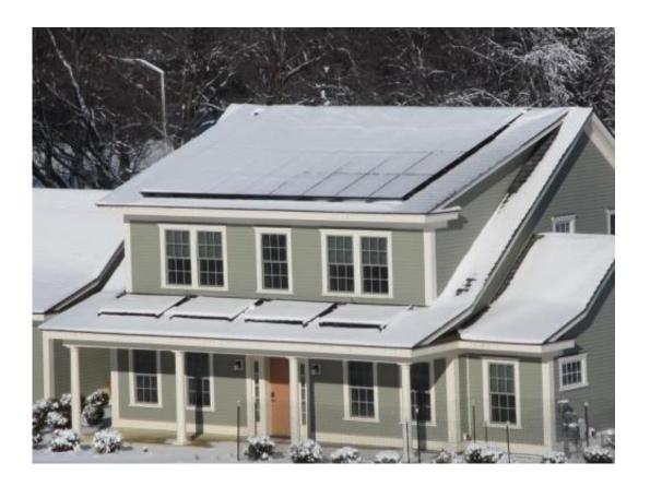
Despite a harsh winter that left the Net-Zero Energy Residential Test Facility's photovoltaic and solar thermal panels covered with snow on 38 days, the energy-efficient house produced more energy than it used over the course of a year. Credit: NIST
