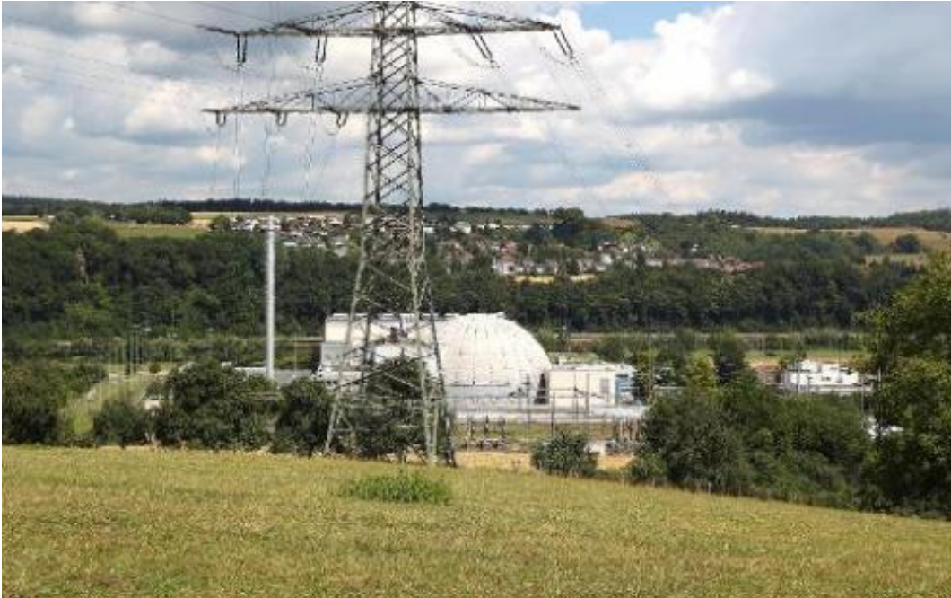
The Nuclear Power Plant in Obrigheim, Germany on July 1, 2014
