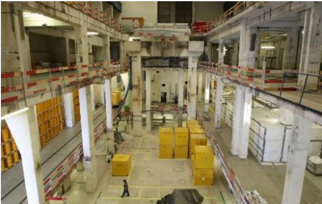
The former machine-hall of the Obrigheim Nuclear Power Plant in Germany
