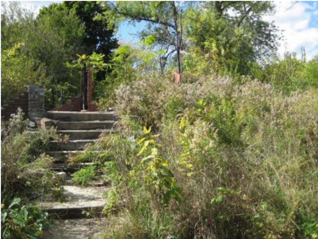
A walkway and steps on a vacant lot in Detroit. Credit: Photo by Daniel Katz
