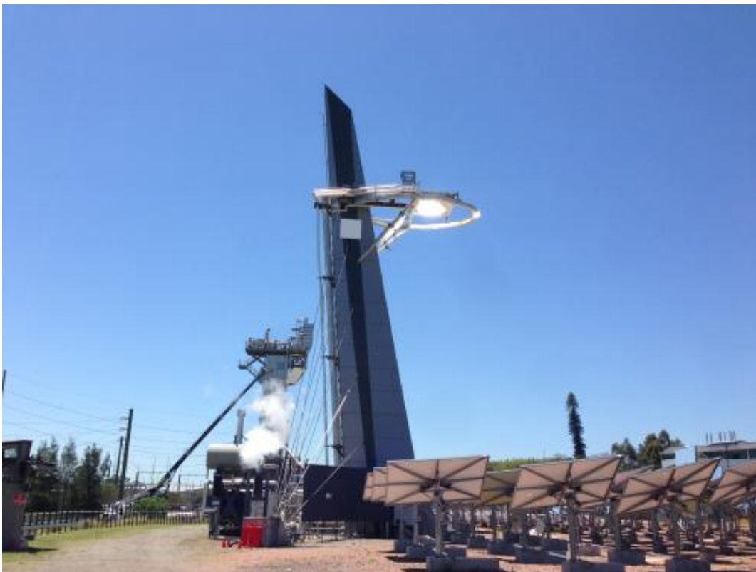
CSIRO Solar tower 1 creating solar steam.
