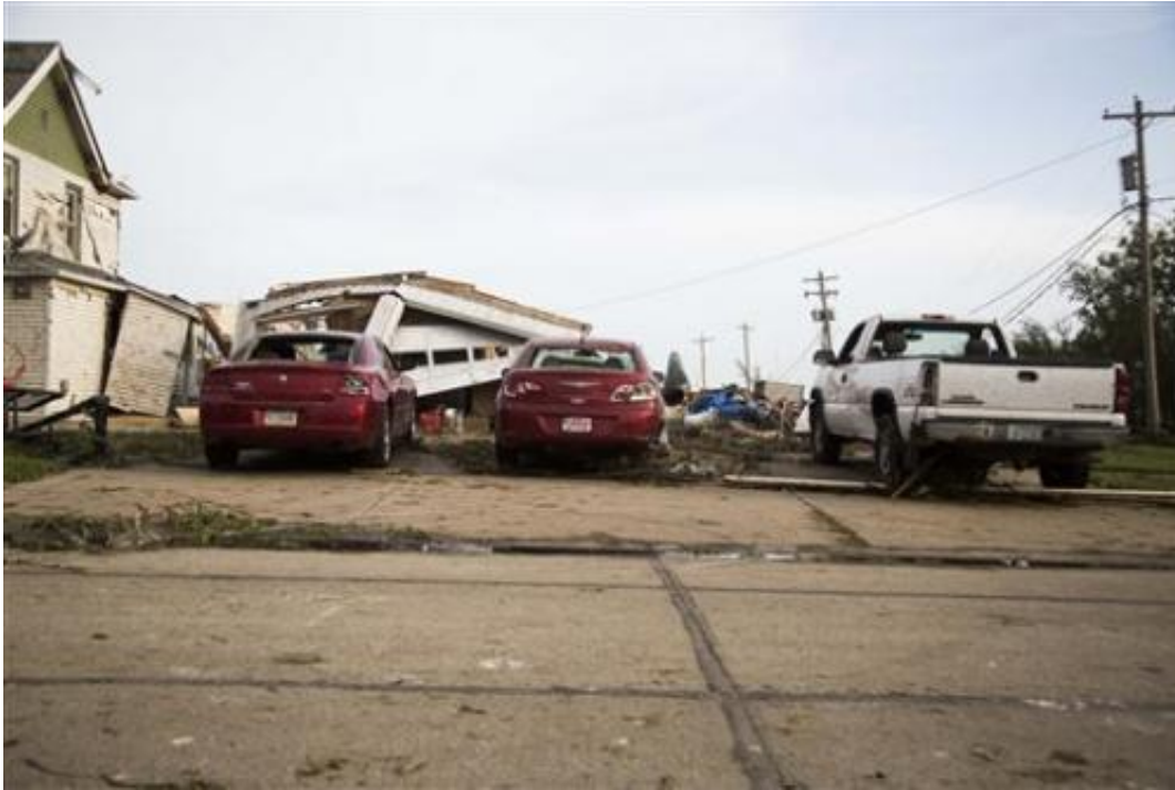
Damaged cars are parked in front of a garage that was torn down by a tornado on Monday, June 16, 2014, in Pilger, Neb. The National Weather Service said at least two twisters touched down within roughly a mile of each other. (AP Photo/The Journal-Star, Stacie Scott)
