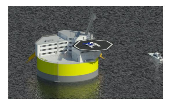
This illustration shows a possible configuration of a floating offshore nuclear plant, based on design work by Jacopo Buongiorno and others at MIT's Department of Nuclear Science and Engineering. Like offshore oil drilling platforms, the structure would include living quarters and a helipad for transportation to the site. Credit: Jake Jurewicz/MIT-NSE
