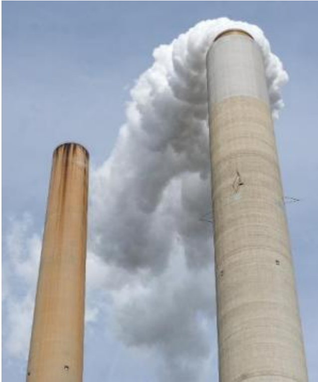
Smoke stacks at American Electric Power's (AEP) Mountaineer coal power plant in West Virginia on October 30, 2009
