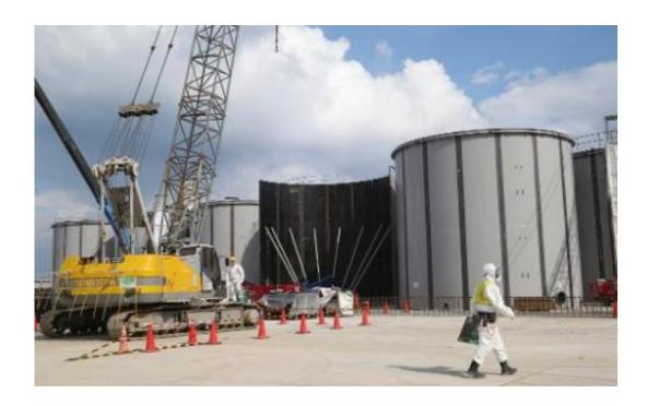
Welded tanks are seen being built above ground at the Fukushima nuclear plant in Okuma, Fukushima Prefecture, on March 10, 2014
