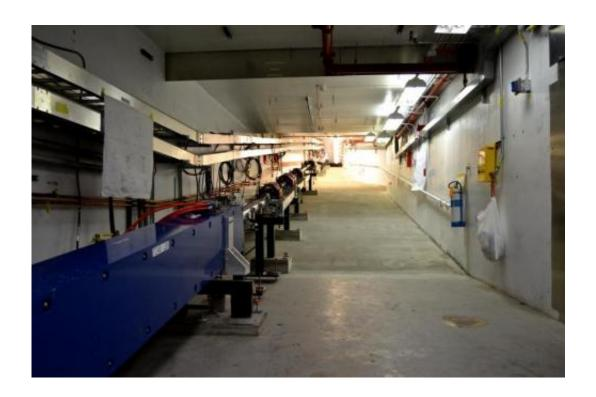
The new beamline connecting Jefferson Lab's CEBAF electron accelerator to its newest experimental area, Hall D, rises 5 meters before entering the Hall D complex. Credit: DOE's Jefferson Lab
