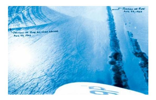
This is a pipeline floatation accident. Taken from the paper by J.S. Damgaard, B.M. Sumer, T.C. Teh, A.C. Palmer, P. Foray and D. Osorio: "Guidelines for pipeline on-bottom stability on liquefied noncohesive seabeds" *Journal of Waterway, Port, Coastal and Ocean Engineering*, ASCE, vol. 132, No. 4, pp. 300-309, 2006. With permission from ASCE. Credit: *Journal of Waterway, Port, Coastal and Ocean Engineering*, ASCE, vol. 132, No. 4, pp. 300-309, 2006. With permission from ASCE.
