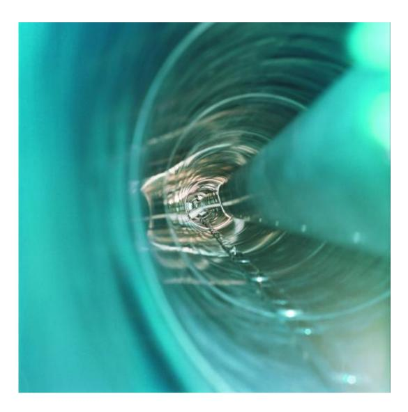
View inside a "pipeline" for electricity: Gas-insulated high-voltage tubular conductor which is suitable in certain cases as an alternative for overhead power transmission lines or high-voltage cables.
