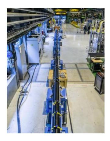
The 20-metre long electrical transmission line containing the two 20 kA MgB2cables. Credit: CERN
