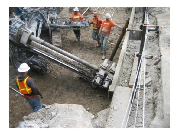
This method could be used in place of having to drill a 'monitoring well' as done in conventional cross-well surveys. Credit: Eric Hodel
