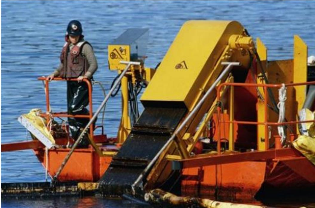
In this April 21, 1989, file photo, a skimmer is used for shoreline oil in Naked Island, Alaska. It collects the oil from off the water surface. The conveyor belt moves the oil onto a barge for storage. Nearly 25 years after the Exxon Valdez oil spill off the coast of Alaska, some damage heals, some effects linger in Prince William Sound. (AP Photo/Rob Stapleton, File)
