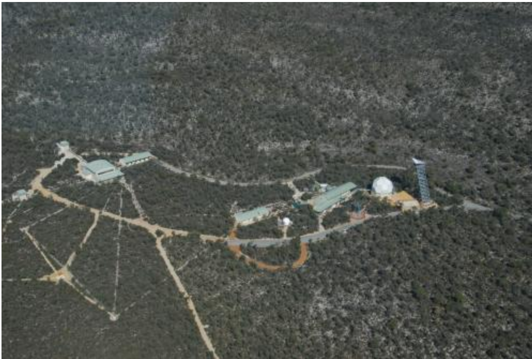
The gravity wave facility at Gingin. Credit: Australian International Gravitational Research Centre.
