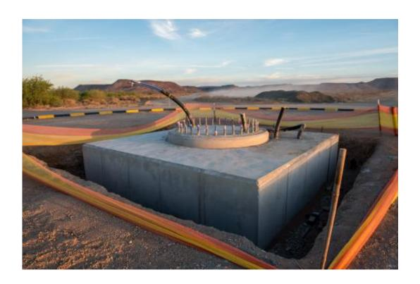
The 64th and final foundation for the MeerKAT telescope antenna was poured yesterday (Tuesday, February 11th, 2014) at South Africa's SKA site in the Karoo. Close to 5 000 m<sup>3</sup> of concrete and more than 570 tons of steel were used to construct the foundations over the last nine months.
