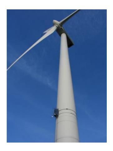
The sensors being attached to the turbine mast. The warning beacons only blink if the radar system detects an airplane. Credit: Fraunhofer FHR
