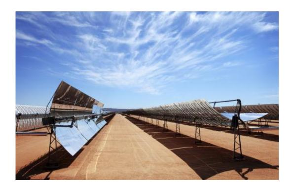
Solar power reflectors collect dust and sand, reducing their energy efficiency—a challenge ORNL researchers are tackling by developing a low-cost, anti-soiling coating.
