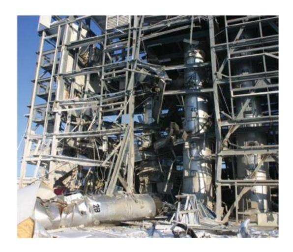
NDK Crystal damage after the incident. The force of the explosion blew out most of the wall panels. Credit: CSB
