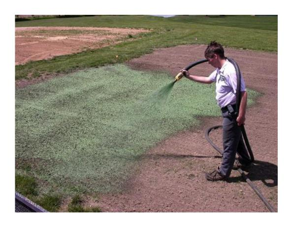
ARS researchers and their industry colleagues tested 10 plant-derived compounds as alternative binders to guar gum in hydraulically applied mulch—hydromulch—like the one being sprayed here.
