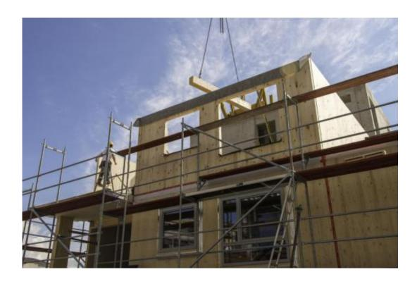
A building in Austria under construction using engineered timber technology.
