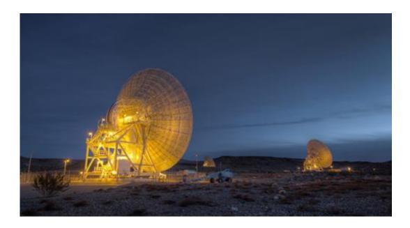
Beam Wave Guide antennas at Goldstone, known as the "Beam Waveguide Cluster." Each antenna is 111.5-feet (34-m) in diameter. They're located in an area at Goldstone called "Apollo Valley." This photograph was taken on Jan. 11, 2012. Credit: NASA/JPL-Caltech
