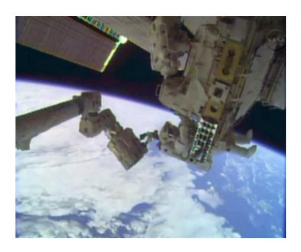
In this image taken from video provided by NASA, astronauts Rick Mastracchio, top, and Michael Hopkins work to repair an external cooling line on the International Space Station on Monday, Dec. 24, 2013, 260 miles above Earth. The external cooling line—one of two—shut down Dec. 11. The six-man crew had to turn off all nonessential equipment, including experiments. (AP Photo/NASA)
