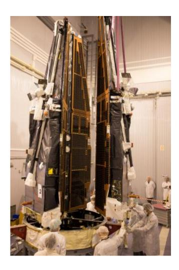
The third Swarm satellite being carefully manoeuvred onto the launch adapter. Packed like sardines, the next major step will be to encapsulate the constellation within the rocket fairing in preparation for launch on 22 November 2013. Credit: ESA–M. Shafiq
