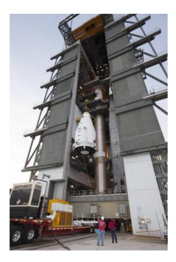
NASA's MAVEN (Mars Atmosphere and Volatile EvolutioN) spacecraft, inside a payload fairing, is hoisted to the top of a United Launch Alliance Atlas V rocket at the Vertical Integration Facility at Cape Canaveral Air Force Station's Space Launch Complex 41. The move and hoisting operations mark another major milestone for the launch team as everything proceeds on schedule to launch Nov. 18, when the Atlas V will lift MAVEN into space and on to Mars.
