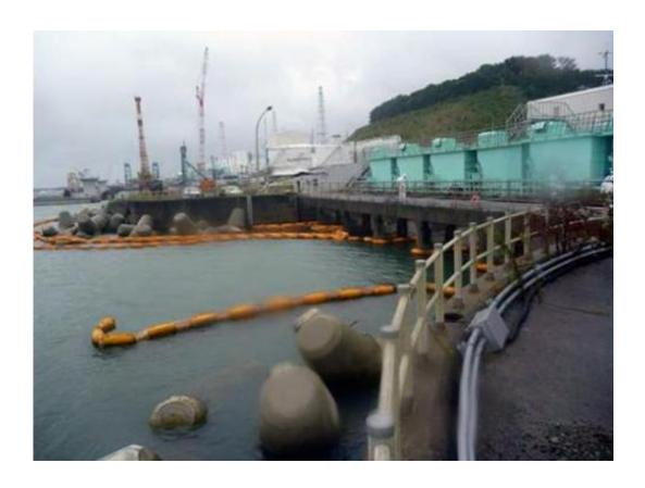
Image provided by TEPCO on September 26, 2013 shows a broken silt fence (yellow floats) at the Fukushima nuclear power plant
