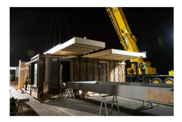
Every good house has a roof. Solar Decathlon Team Austria has also heard of this wisdom – which is why LISI received her "headgear" today. Four ceiling modules make up the roof – crowned by sparkling photovoltaic modules. Deep into the night, the crane placed one module at a time.
