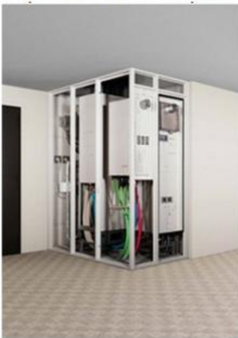
Pipe shaft with doors open
