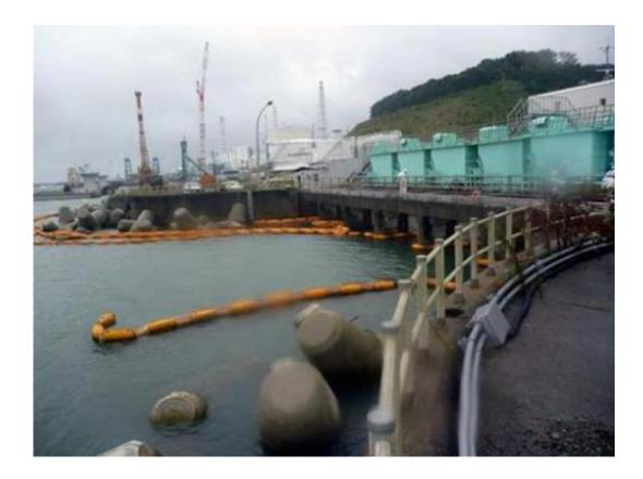
A silt fence, a device to trap sediment before water flows into the sea, at the stricken Fukushima nuclear power plant on September 26, 2013
