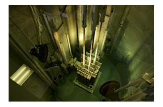
NRAD is a small, water pool-type 250-kW Training, Research, and Isotope reactor designed and manufactured by General Atomics (TRIGA).
