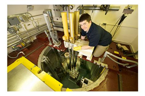
INL's NRAD reactor allows researchers to examine the insides of nuclear fuel and other materials similar to the way X-rays are used. Here, a technician poses above the reactor when its cover had been removed for a maintenance outage in 2010.
